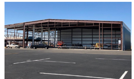
Fox Hangar Construction
