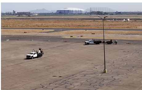
Crack Seal
