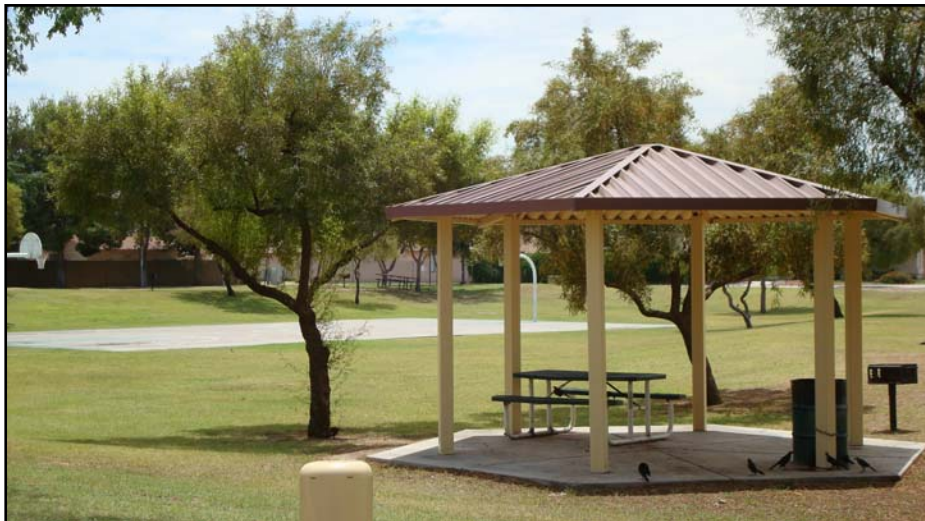
Project Name: Pasadena Park Source: DIF Fund #: 1520 Project #: 70454
