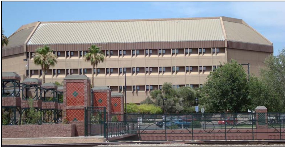
Project Name: City Hall – HVAC System Funding Source: G.O. Bond Fund #: 2080 Project #: 77504
