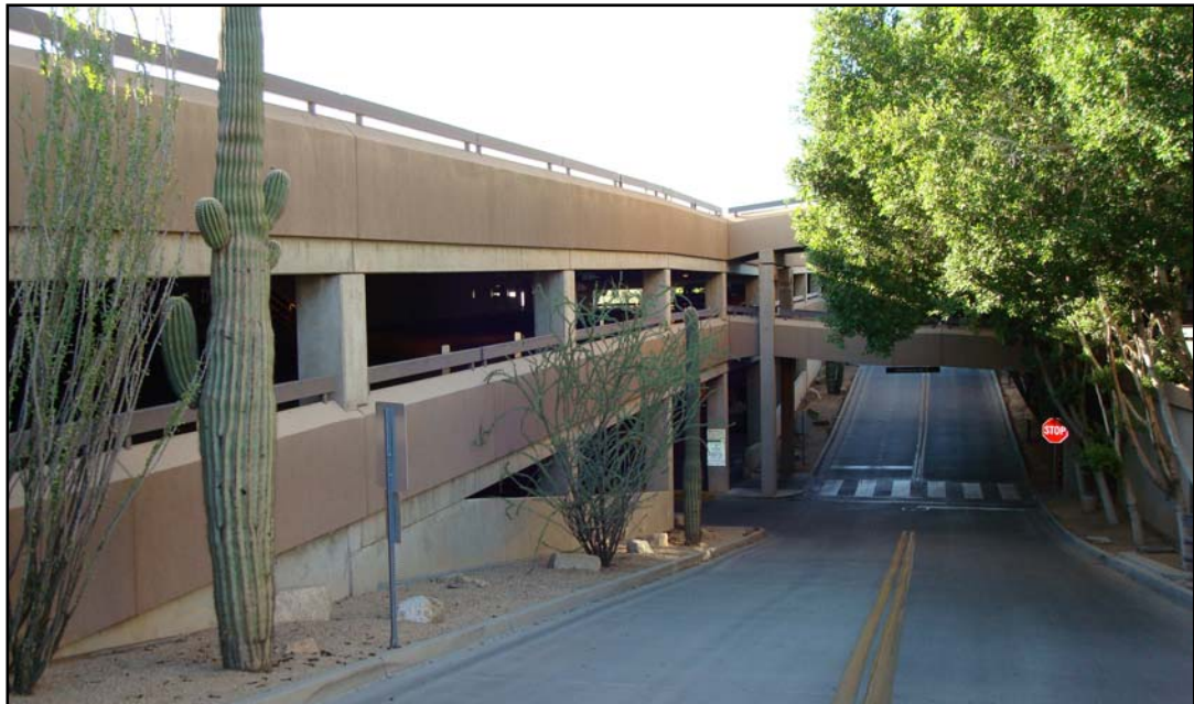
Project Name: City Hall Parking Garage Funding Source: G.O. Bond Fund #: 2080 Project #: T1160
