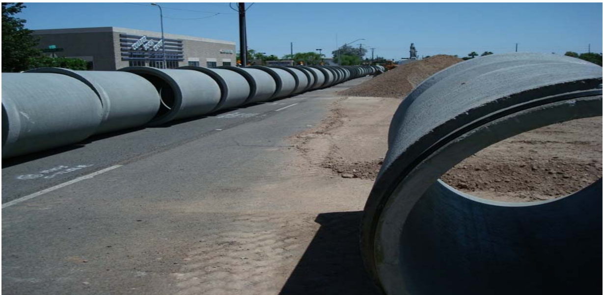
59 th Ave Storm Drain Project
