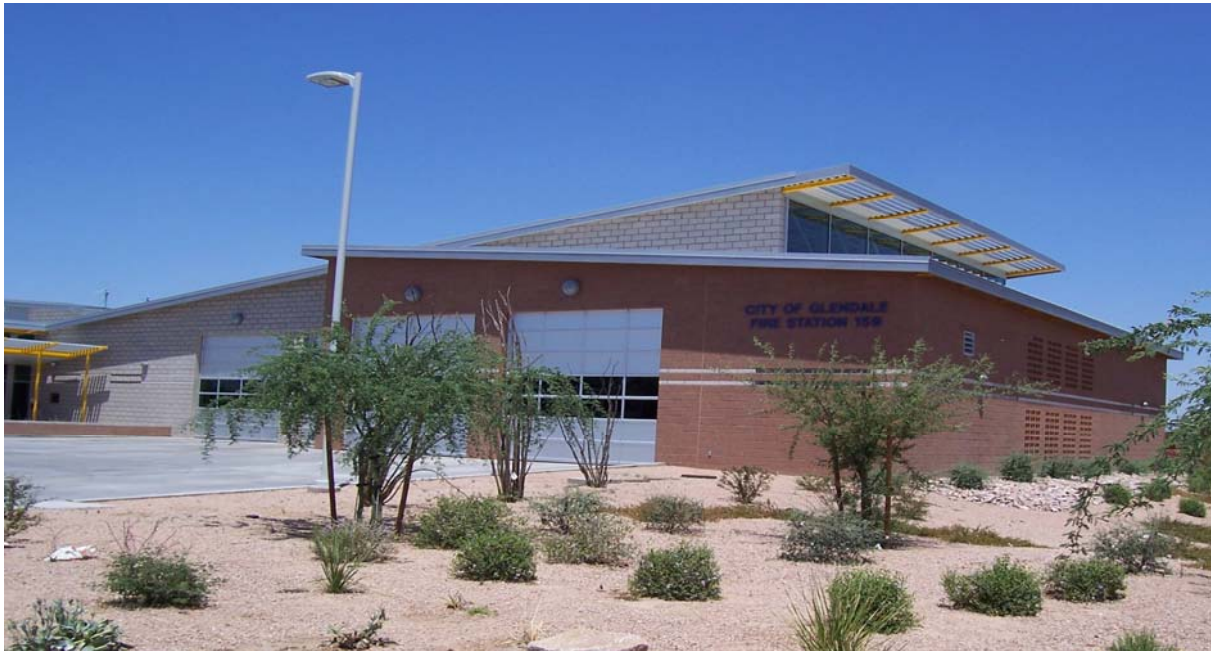
Glendale Fire Station 159
