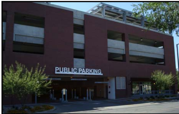
Project Name: Downtown Parking Structure Funding Source: G.O. Bond Fund #: 1980 Project #: 68113
