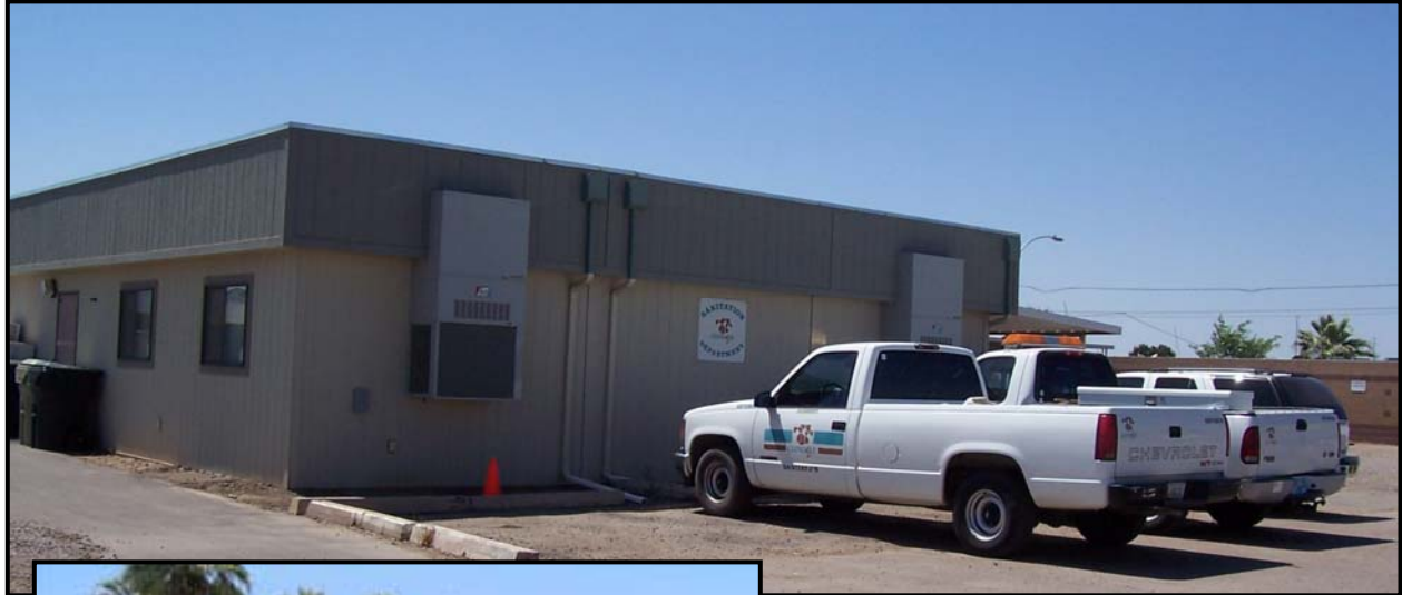
Project Name: Sanitation Office Trailer Fund #: 2480 Project #: T2411 Picture Note: Sanitation's current office trailer.
